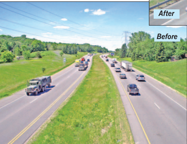
From Excelsior Boulevard, looking north.
