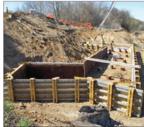
(CLOCKWISE FROM THE TOP LEFT) Pile driving for the Orchard Road bridge, concrete forms for the bridge abutment, excavation for utility relocation, and crews installing new valves on a water main.
