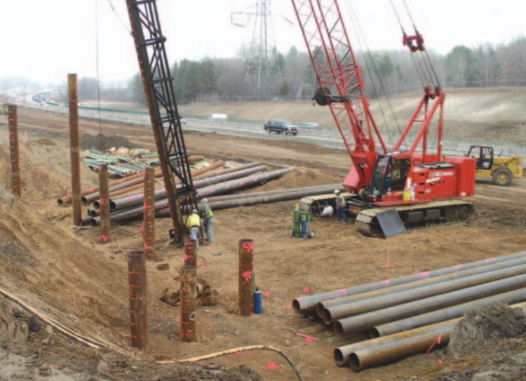
(CLOCKWISE FROM THE TOP LEFT) Pile driving for the Orchard Road bridge, concrete forms for the bridge abutment, excavation for utility relocation, and crews installing new valves on a water main.
