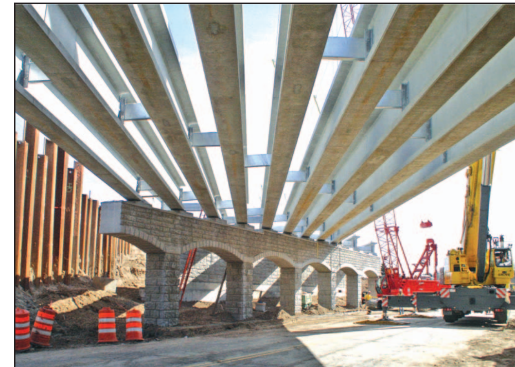
Concrete beams for the new I-494 southbound bridge over Baker Road.
